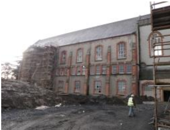
Demolition of Old St.Joseph's School.. 2012
